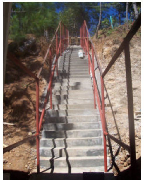
Stairway to the Engineering department under construction. A canopy was installed for convenience of passerby during rainy season.
